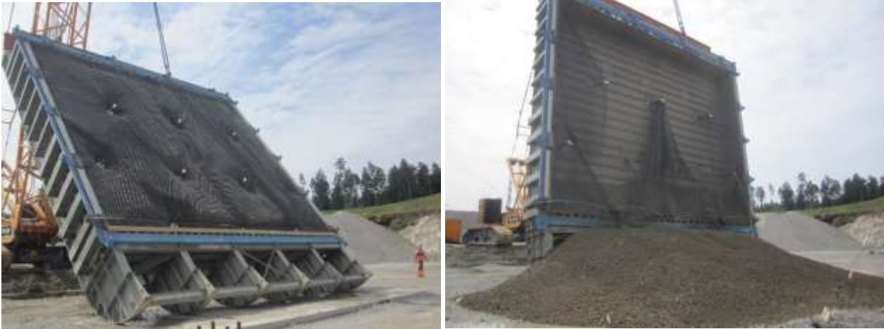
Figure 9. Test No. 11 TECCO® G65/3 + P33, nail grid 3.5×3.5m, sandy gravel 0–63 mm, \alpha = 53^\circ , first superficial movements (left) and at failure at \alpha = 80^\circ (right).
