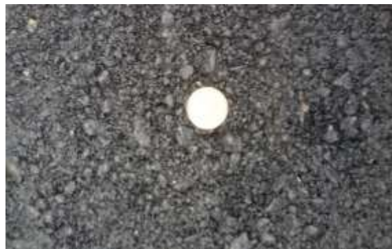
Figure 7. Asphalt Concrete – Step 2
