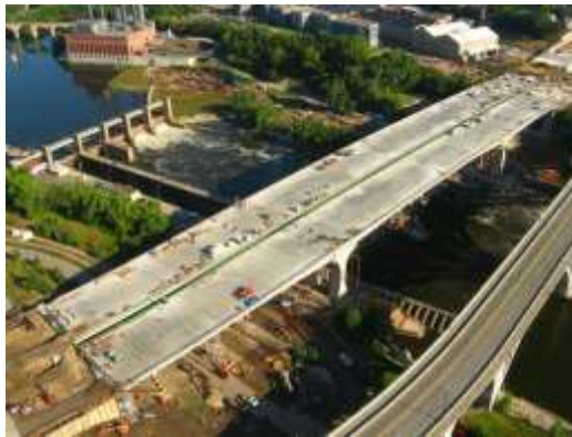
Figure 2: New I35W Bridge in Minneapolis
