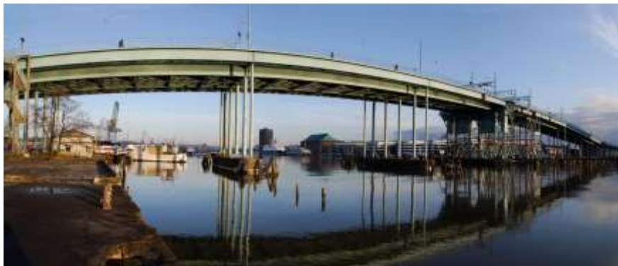
Figure 10: View to nearly one kilometer long Götaälvbron Bridge.
