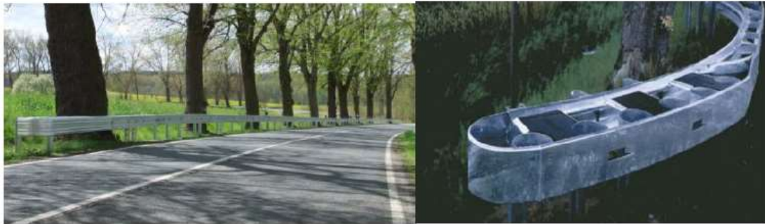
The ends of the guardrails should be rounded
