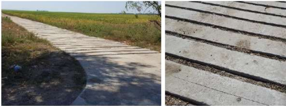
Agricultural access road from ribbed concrete (expensive but most efficient solution, example from Serbia)
