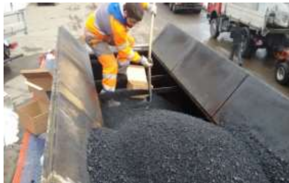
Figure 6. Asphalt Concrete – Step 1
