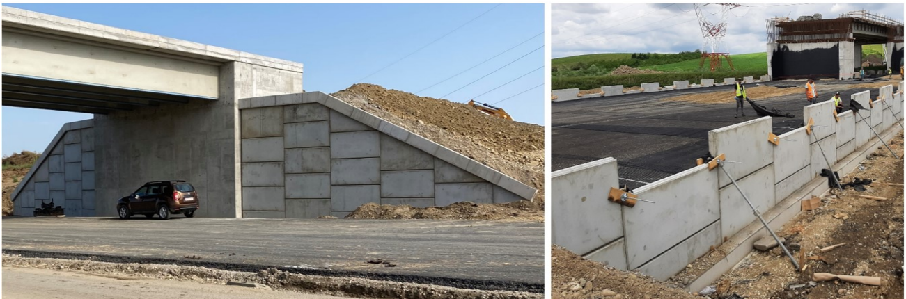
Figure 6. Discrete concrete panels installed as an active facing (Targu Mures, Romania)
