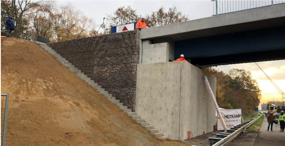
Figure 8. View of one of the considered abutment after completion
