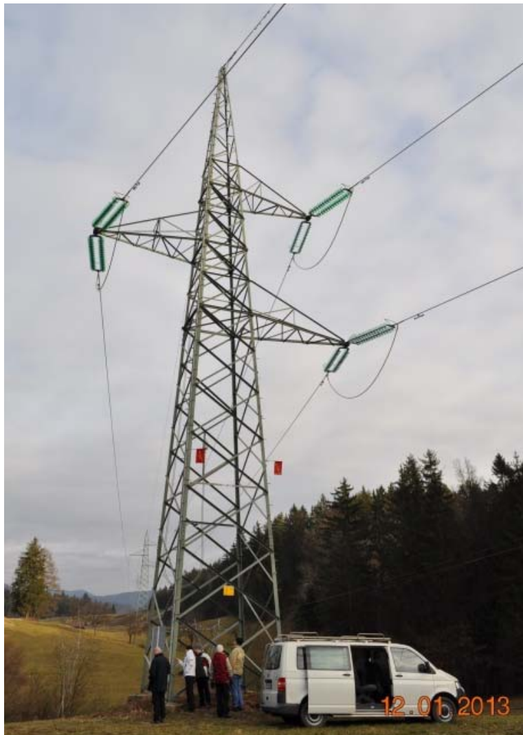
FIGURE. 1: Real transmission tower structure
