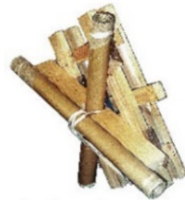
Fig. 5 Fragment of a joint of a grid shell of Japan Pavilion in Hanover
