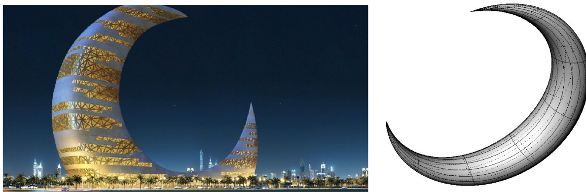
Fig. 9 – The half a cone harmonic equivalent – from left to right, Crescent Moon Tower in Dubai, top-skewed view, respectively
