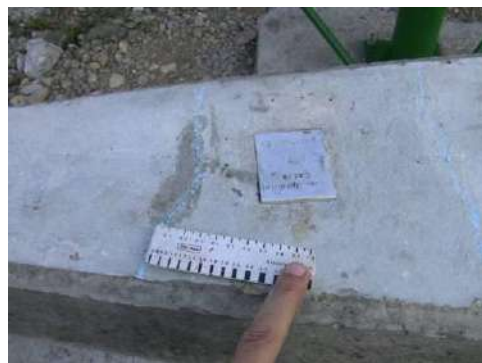
Figure 7 – Measuring of dilatations and cracks
