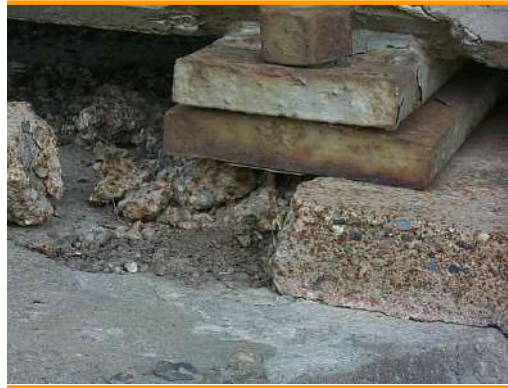
Figure 11 - Damaged support condition
