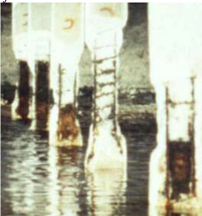
Figure 8 - Damaged concrete and wood piles
