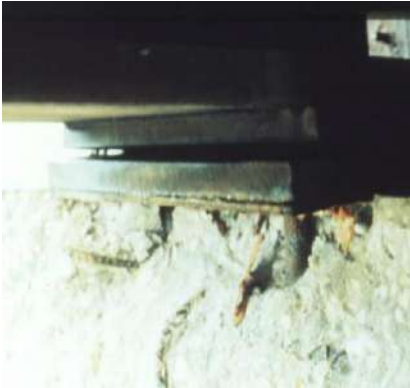
Figure 11 - Damaged support condition
