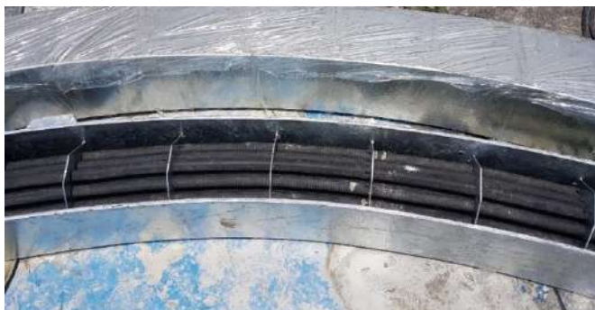
Figure 5 – Saddle steel formwork with recesses bars installed
