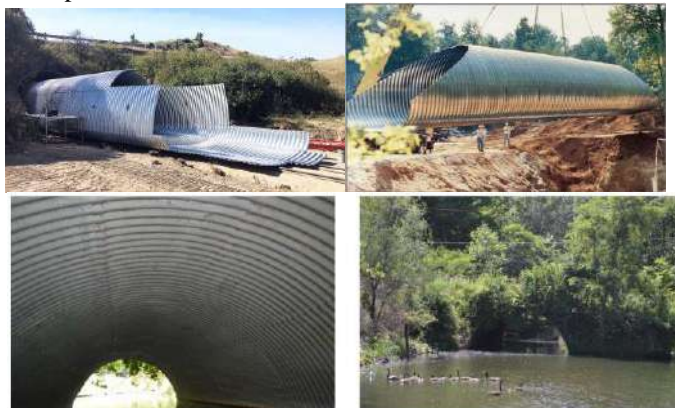
Figure 8 – Upper: steel corrugated pipe installation (Contech catalogue); lower: typical steel corrugated pipe culverts in the U.S.A
