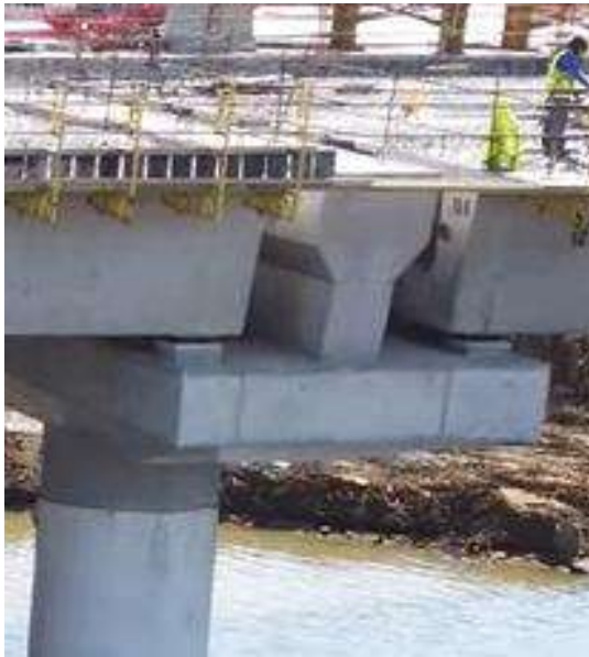
Figure 6 – Built pier support detail
