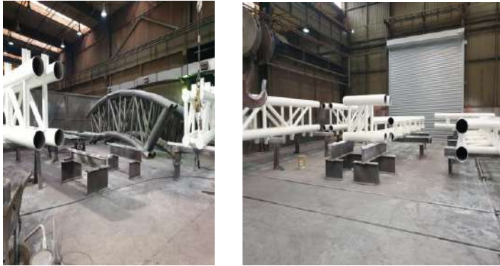
Figure 11 - Application of anti-corrosion protection
