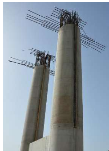
Figure 12 – The pillar with 8 m high split part
