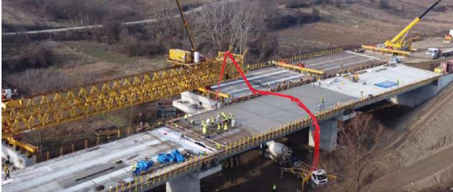
Figure 4 – Longitudinal view of the bridge at km8+519 (under construction)
