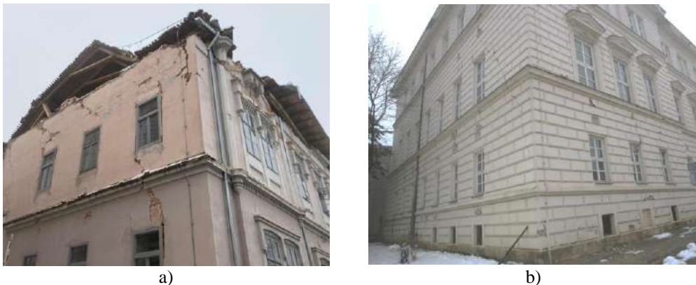
Figure 3 – Damage of URM schools in Petrinja, Croatia: a) exterior damage of the First school building and b) inclined shear cracks in the walls of the Petrinja High School
