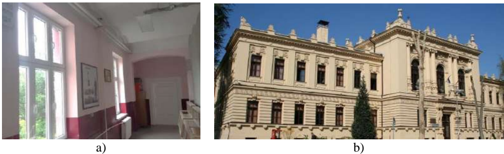
Figure 8 – URM schools in Serbia: a) Primary School Milisav Nikolić in Malo Crniće and b) High School in Valjevo
