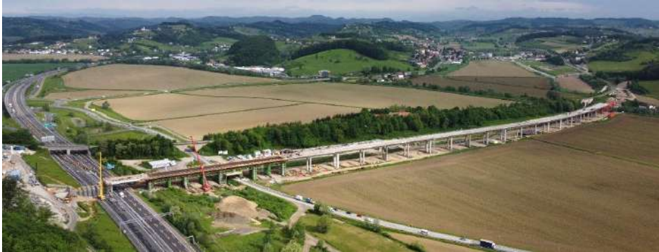
Figure 13 – Concreting of 112 m segment and almost finished structure (spring 2022)
