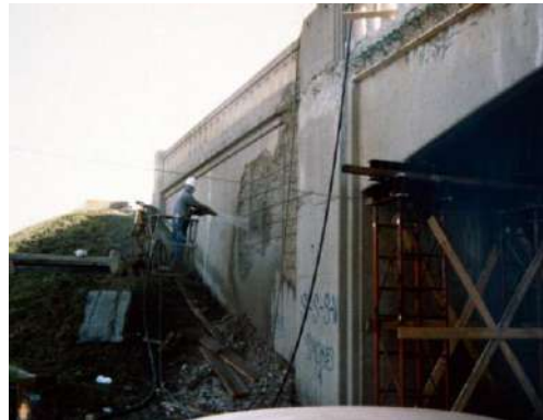
Figure 7 - Shotcrete repair of bridge abutment
