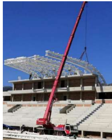
Figure 16 - Lifting of main girders
