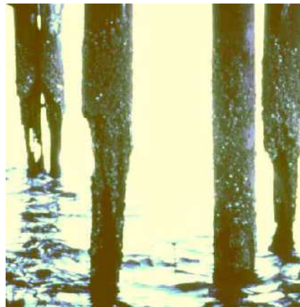
Figure 8 - Damaged concrete and wood piles
