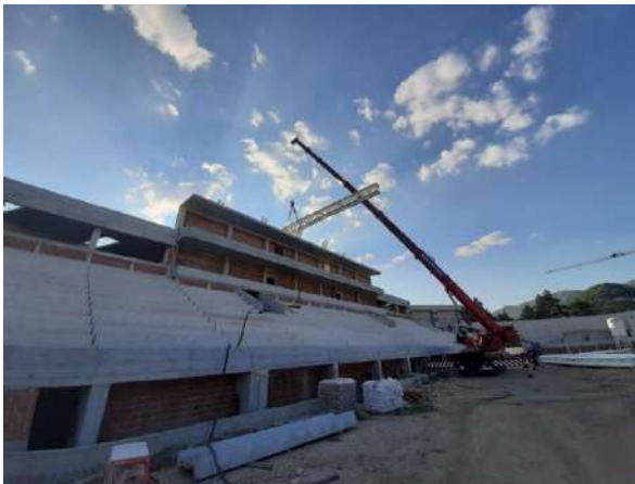
Figure 15 - Lifting of main girder N1
