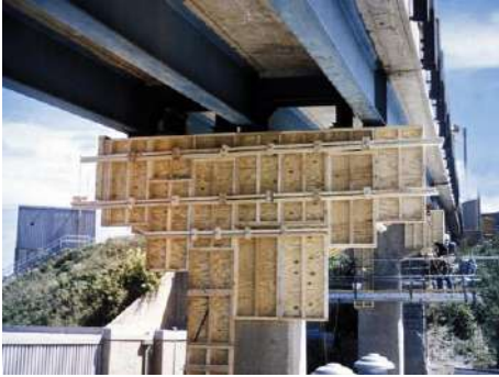
Figure 3 - Forms in place and completed repair
