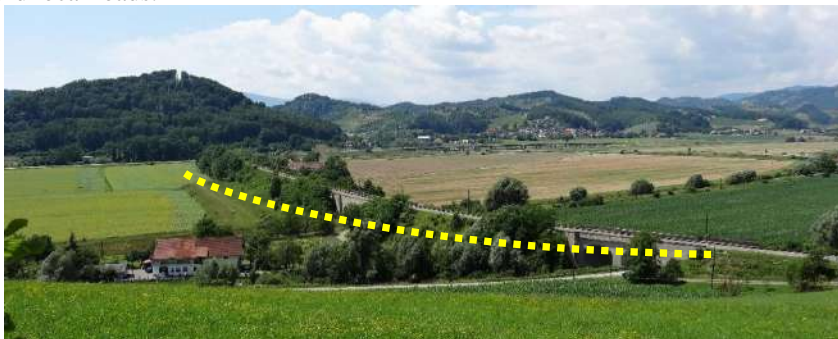
Figure 2 – The existing railway line on the dyke and the new route
