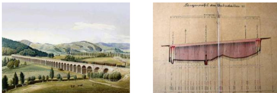
Figure 1 – The former railway viaduct over the Pesnica River Valley dated 1846; left: artistic representation; right: section of the longitudinal profile plan
