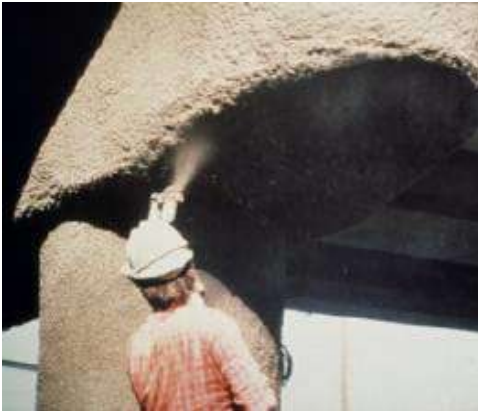
Figure 6 - Shotcrete repair of bridge pier
