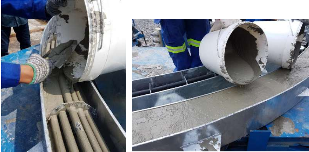
Figure 6 – Saddle UHPFRC pouring
