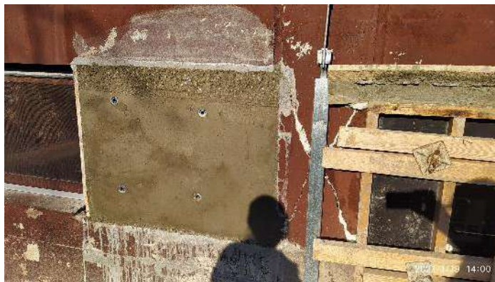
Figure 10 – RC segment after pouring of concrete
