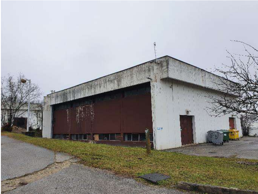
Figure 3 – View of the building from the south-east corner
