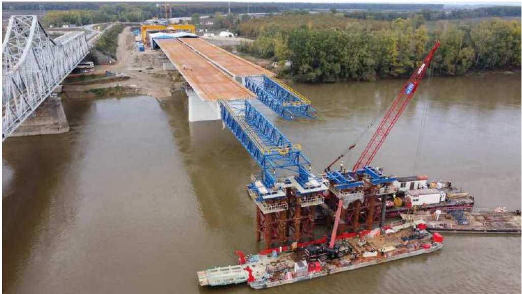
Figure 11 - First bridge reaching the temporary pier in the river
