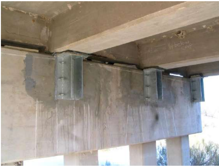
Figure 12 – Bearing seat retrofit
