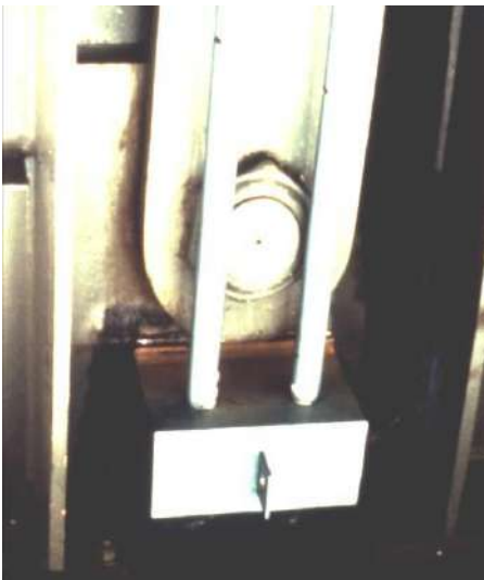
Figure 14 - Pin-hanger retrofit
