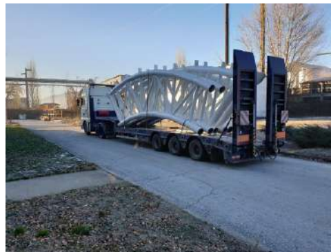
Figure 13 - Transport of steel structure assemblies
