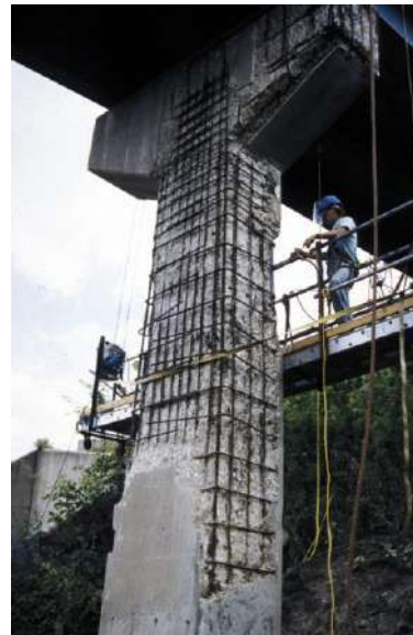
Figure 2 - Removal of deteriorated concrete
