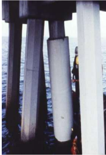
Figure 9 - Concrete pile jackets
