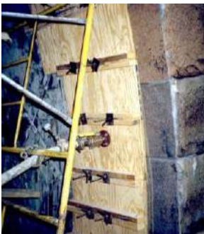
Figure 5 - Form and pump equipment and completed repair
