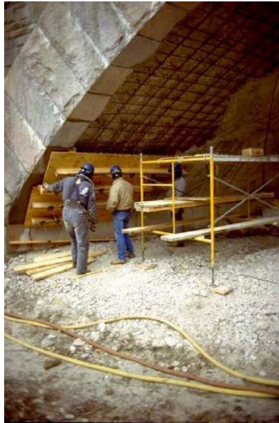
Figure 4 - Preparation of reinforcing steel and concrete formwork
