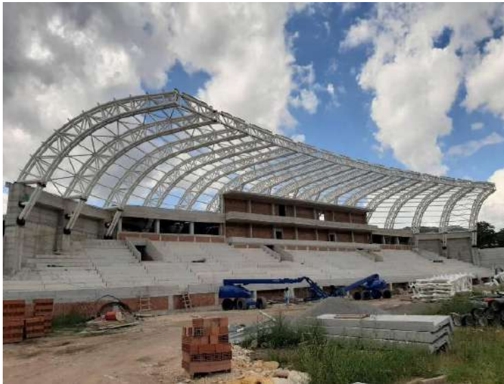
Figure 17 - Erected steel structure
