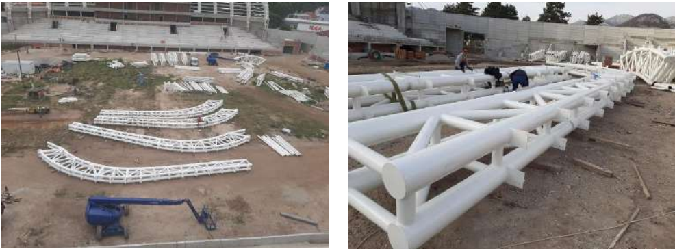
Figure 14 - Preparation of main girders on construction site
