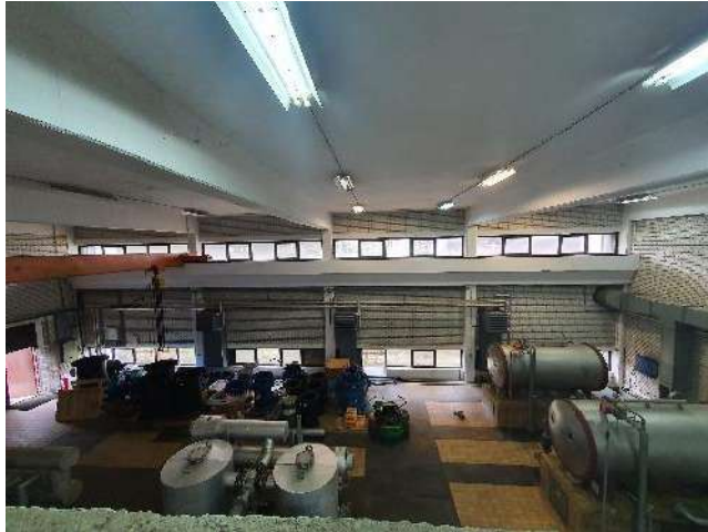
Figure 5 – Interior of the building, looking to the south
