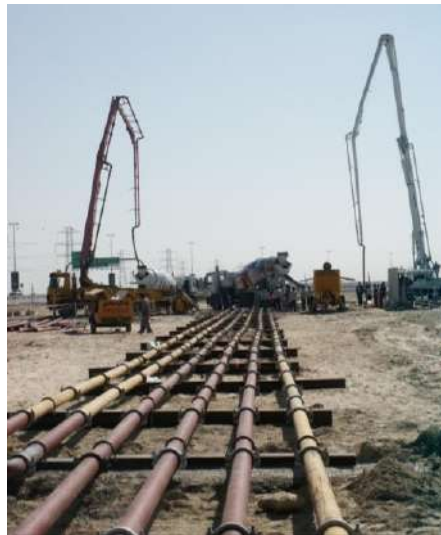
Figure 10 – Burj Khalifa Concrete Pumping Test (SOM)
