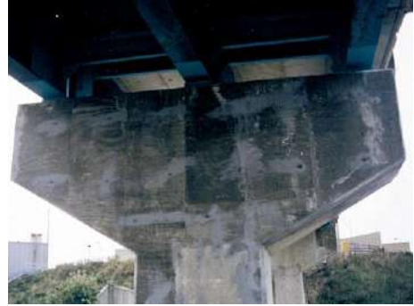
Figure 3 - Forms in place and completed repair
