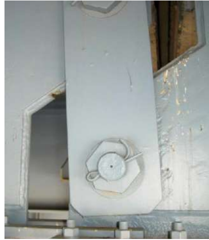
Figure 13 - Wear, fatigue, corrosion of pin/hanger
