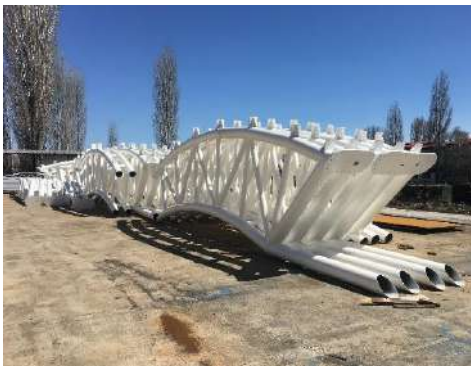
Figure 12 - Assemblies of steel structure prepared for transport
