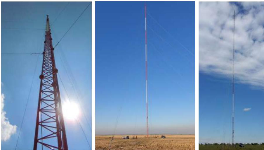
Figure 1 - Installed guyed masts of 120.78m, 160.00m and 126.30m height, respectively (source: NETInvest Engineering and Consulting Solutions)
