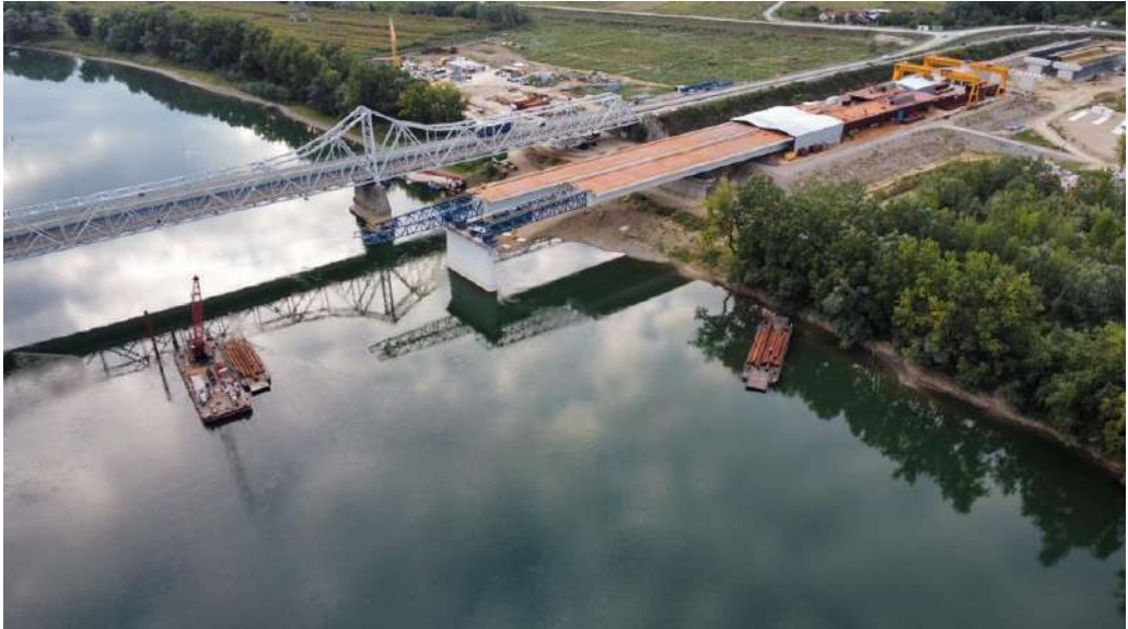
Figure 9 - Beginning of the launching, one bridge launched 30 m
