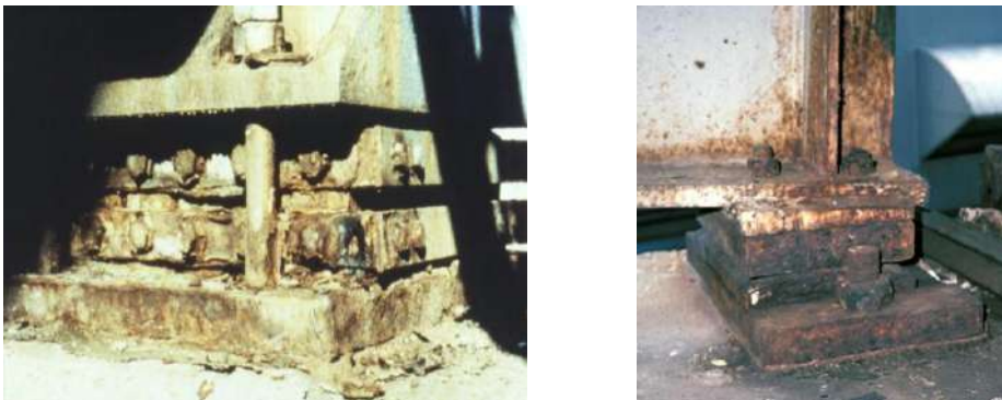
Figure 10 - Frozen bearings
